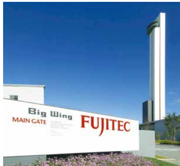
Big Wing (Group Headquarters in Japan, Elevator Plant)
