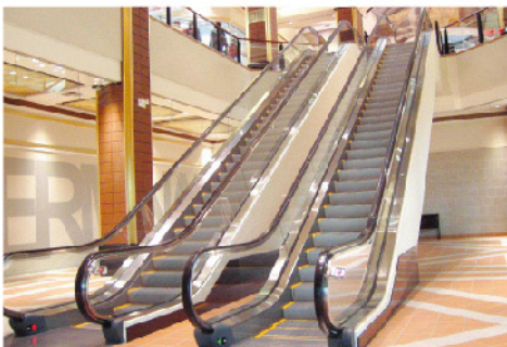
Atlantic Terminal New York, USA
